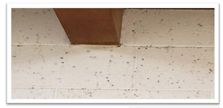
turned on in October, the water within the ductwork caused an increase in the humidity within the church. The humidity was as high as 85%.
