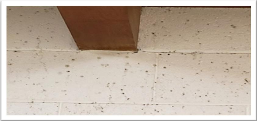
The out-of-control humidity caused severe mold growth within the front foyer, office and in the stairwell. An analysis of the air quality within the church showed mold spores up to 100 times the safe limit. With such dangerously high mold spore levels, St. Peter's was forced to close its doors until the problem could be resolved and the church deemed safe to reenter.
