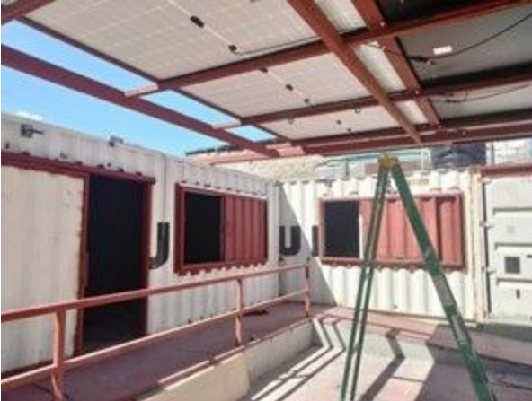
Solar panels provide power and shade for the retrofitted containers at the St. Vincent's Medical Center in downtown Port-au-Prince.
